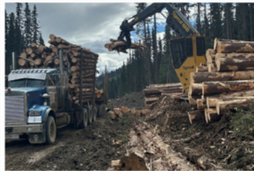
LOGGING & ROW CLEARING
